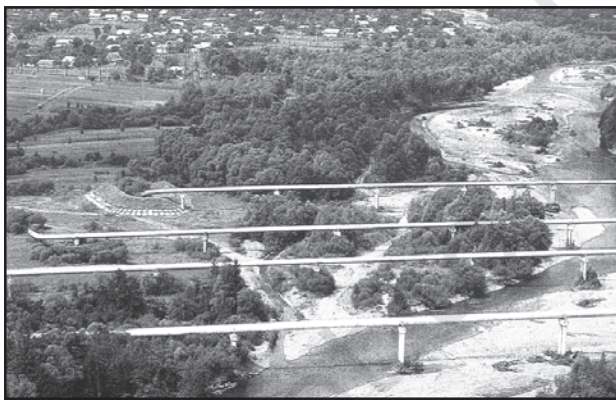
Fig. 7.17: Pipelines transporting natural gas in Ukraine
